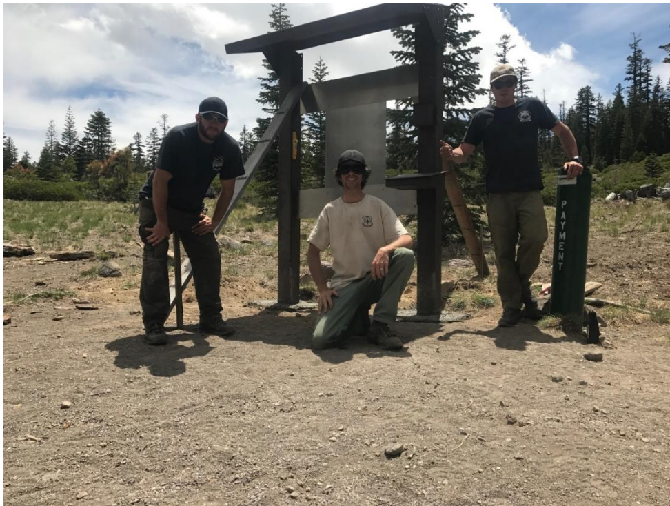
Left to right: Paul Moore, Nick Meyers and Forrest Coots pose in front of a newly installed trailhead kiosk at Northgate. These all steel kiosks were installed at Sand Flat, Old Ski Bowl, Clear Creek, Brewer Creek, Northgate and Whitney Falls trailheads. They look great and should last a LONG time. A grant (associated with the summit pass fees generated) and matching funds from local sponsors funded this project. A big thanks to The 5 th Season, Berryvale, Shasta Mountain Guides, Sierra Wilderness Seminars, The Sierra Club Foundation and Shasta Base Camp.
